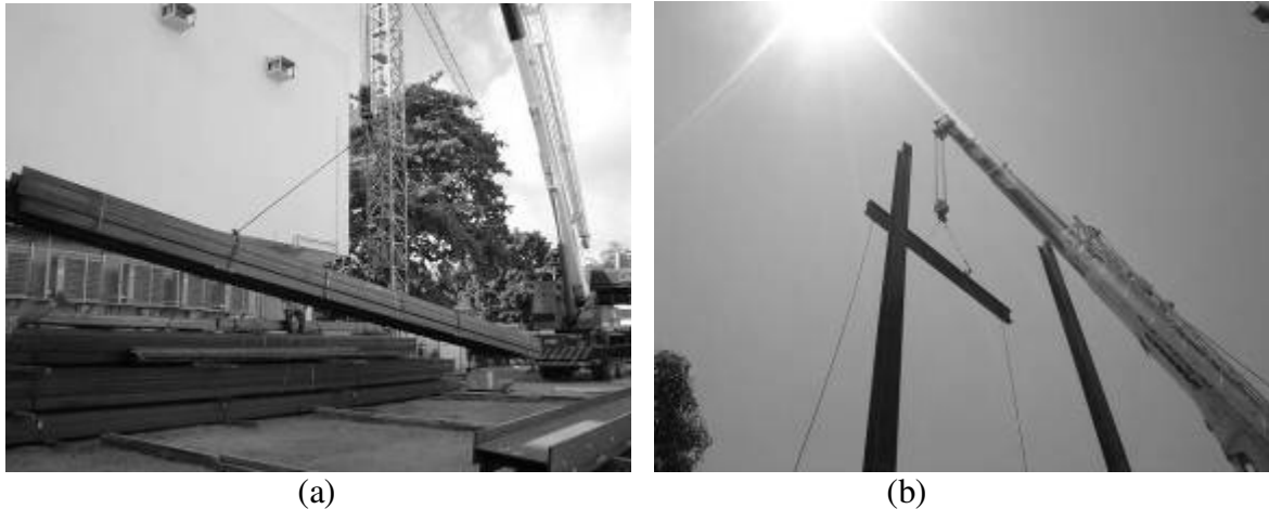
Figure 1 - Displacement of heavy profiles (a) and Assembly of metallic beam (b)
