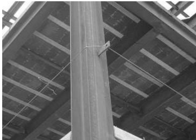
Figure 2 - Steel handles settled in accessories welded in the pillar
